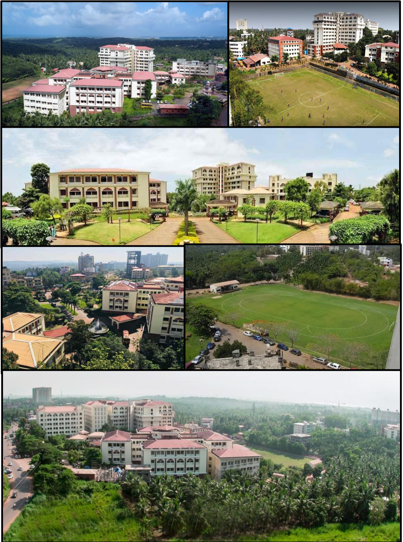
Eco-friendly Campus Yenepoya (Deemed to be University), Mangalore, Karnataka - Greenery view
