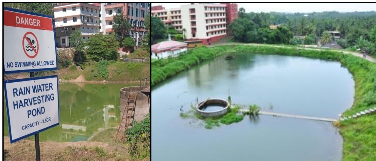
Rain water harvesting pond in Yenepoya (Deemed to be University), Mangalore, Karnataka
