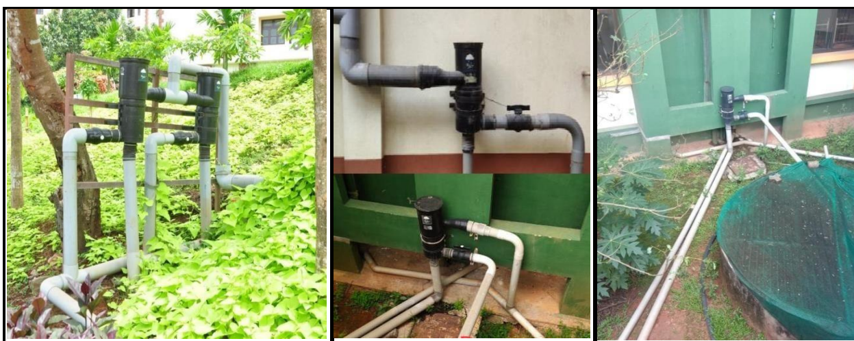
Roof rainwater harvesting units for recharging borewells and for open wells in Yenepoya (Deemed to be University), Mangalore, Karnataka
