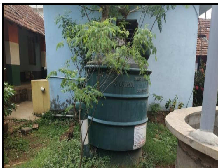
Biogas plant facility in Yenepoya (Deemed to be University), Mangalore, Karnataka.
